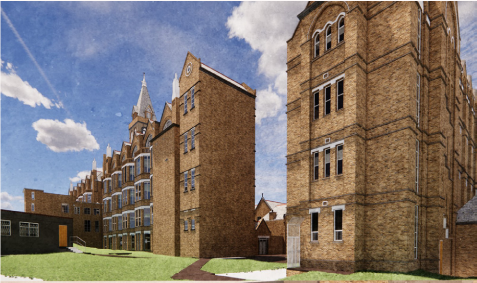
WEST FAÇADE EXISTING VIEW
