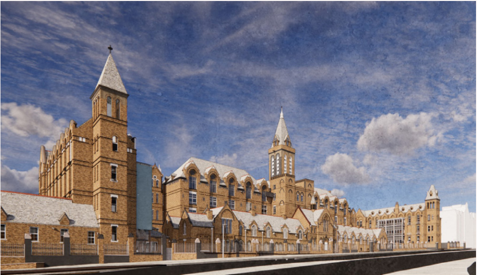
EXISTING VIEW FROM ARCHWAY ROAD
